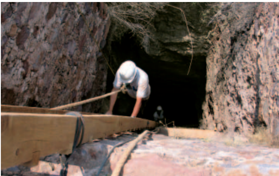
Access and cleaning of old shafts at San Celso
